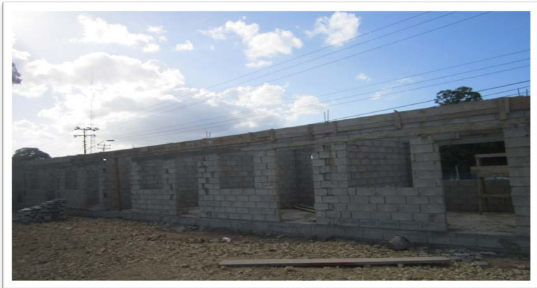
Vendors Booths under construction at Irwin Park, Siparia
