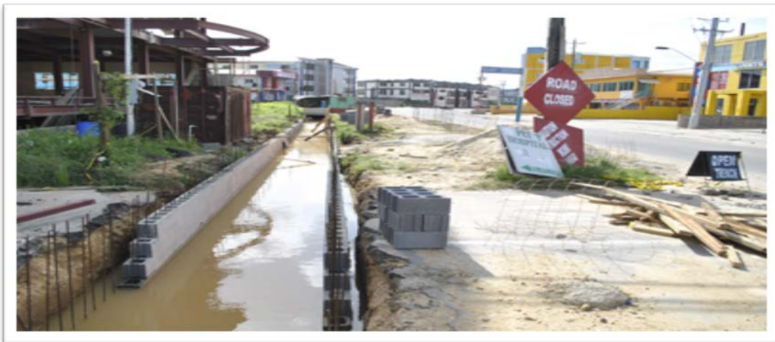
Development of Ramsaran Street Boulevard underway
